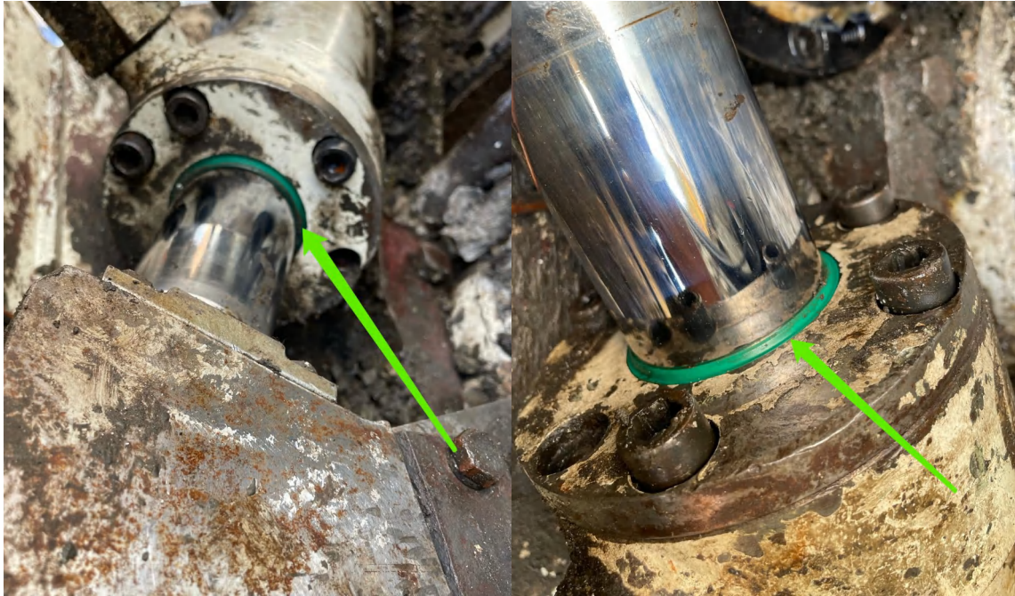
Hydraulic cylinder seal replacement
