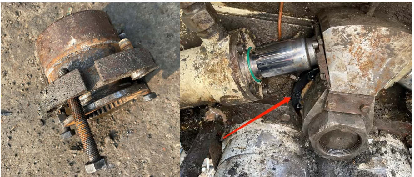
Hopper small end and seal ring replacement
