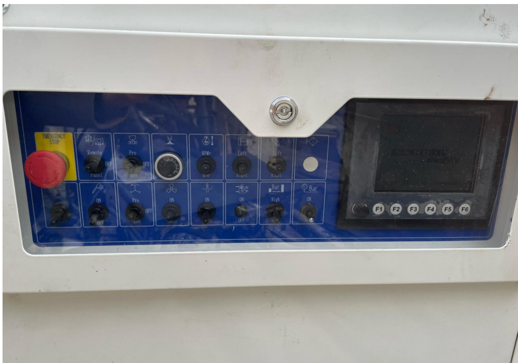
Electrical control cabinet replacement
