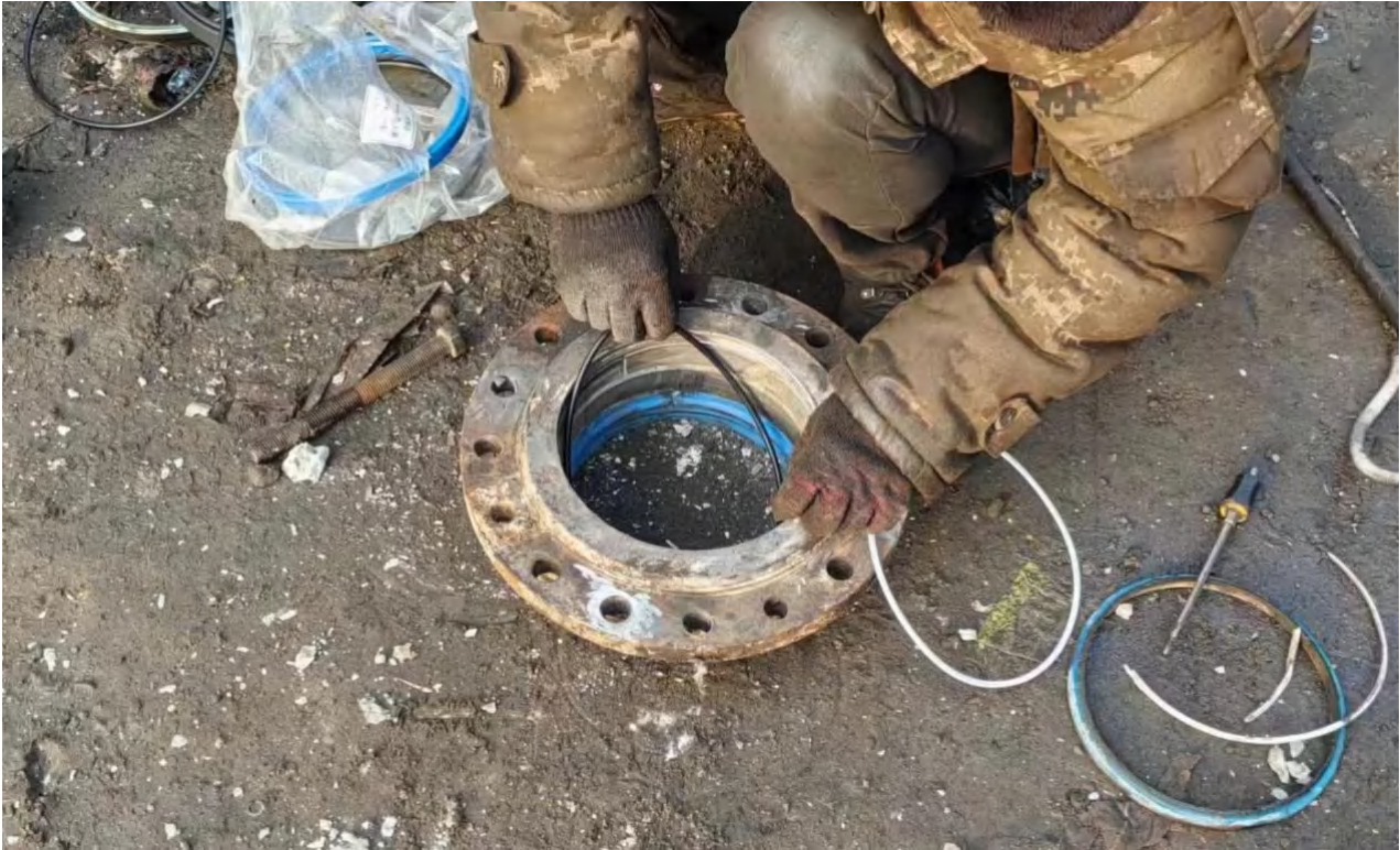
Hopper big end seal replacement
