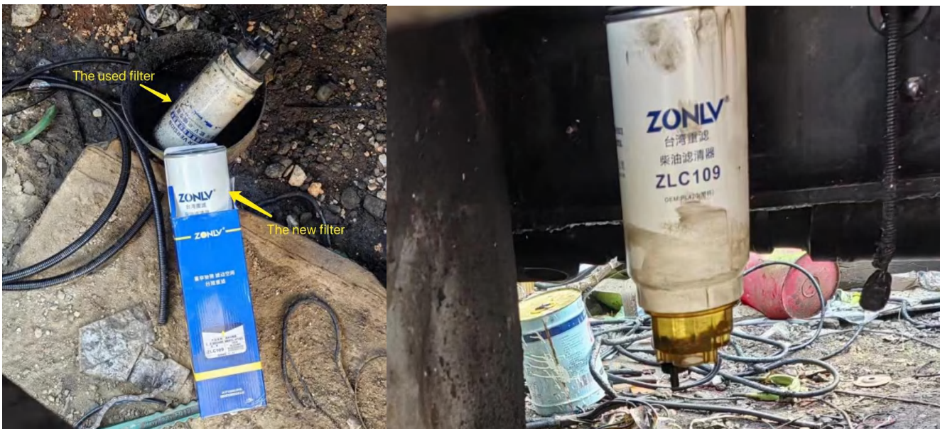
Engine oil-water separator filter replacement
