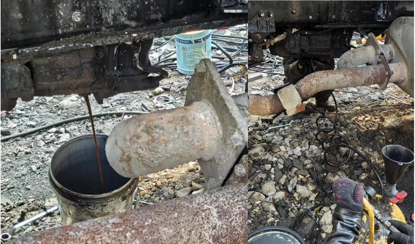
Transmission gear oil replacement
